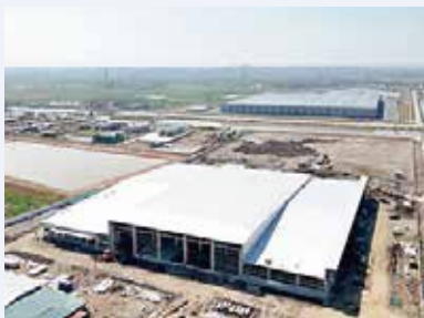
▲ Scenes of construction (October)
